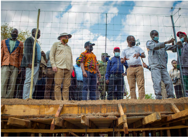
Page 3 communities construct park fence
